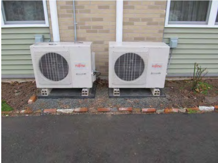
Typical exterior condenser units for ductless mini-split heat pump systems installed in all units during 2012
