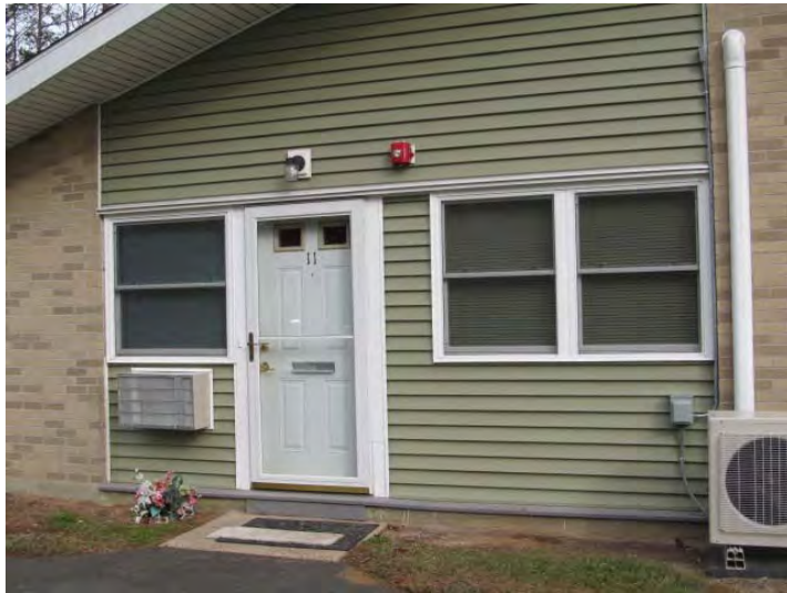
New vinyl siding, windows, entry doors, and storm doors installed as part of a renovation scope of work completed in 2009
