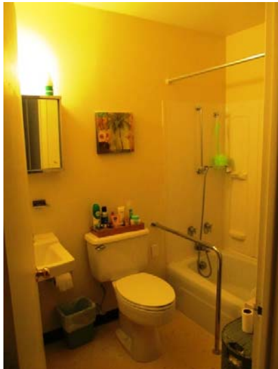
Typical finishes and fixtures in unit bathrooms – Note bathtubs/showers are not equipped with contemporary anti-scald mixing valve assemblies
