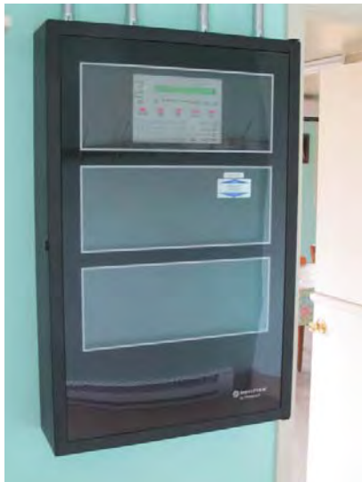
Fully addressable fire alarm control panel for monitoring and supervision of common area and in-unit end devices – No problems observed or reported
