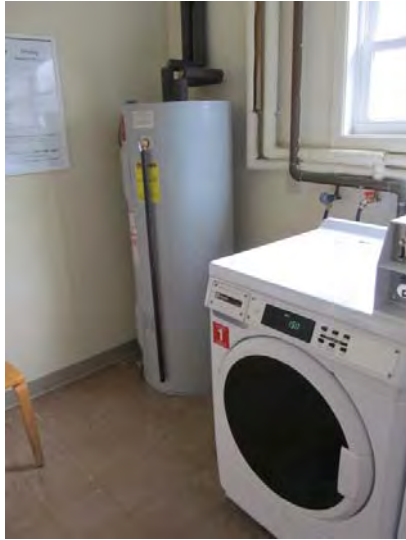
Newer electric domestic hot water tank serving community building
