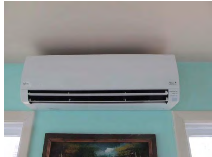
Interior wall-mounted section of ductless mini-split system heat pump at community building
