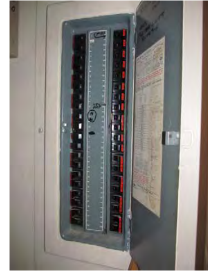
Electrical load center at community building is comprised of a Stab-Lok circuit breaker panel – This brand of equipment has a history of failure and service parts are no longer available
