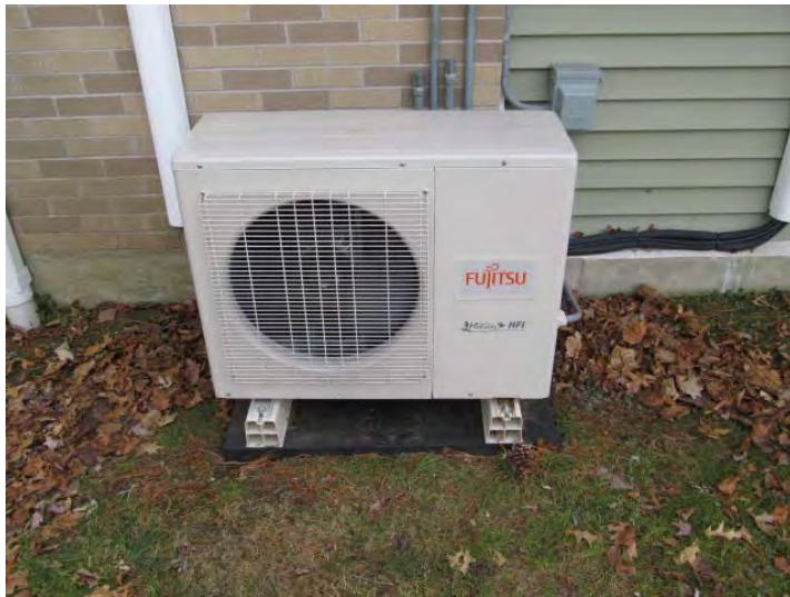
Exterior condenser unit for ductless min-split heat pump system installed at community building in 2012
