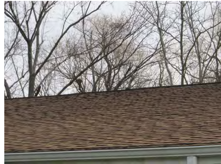
Renovation work completed in 2009 also included installation of new architectural-style shingles on all roof surfaces
